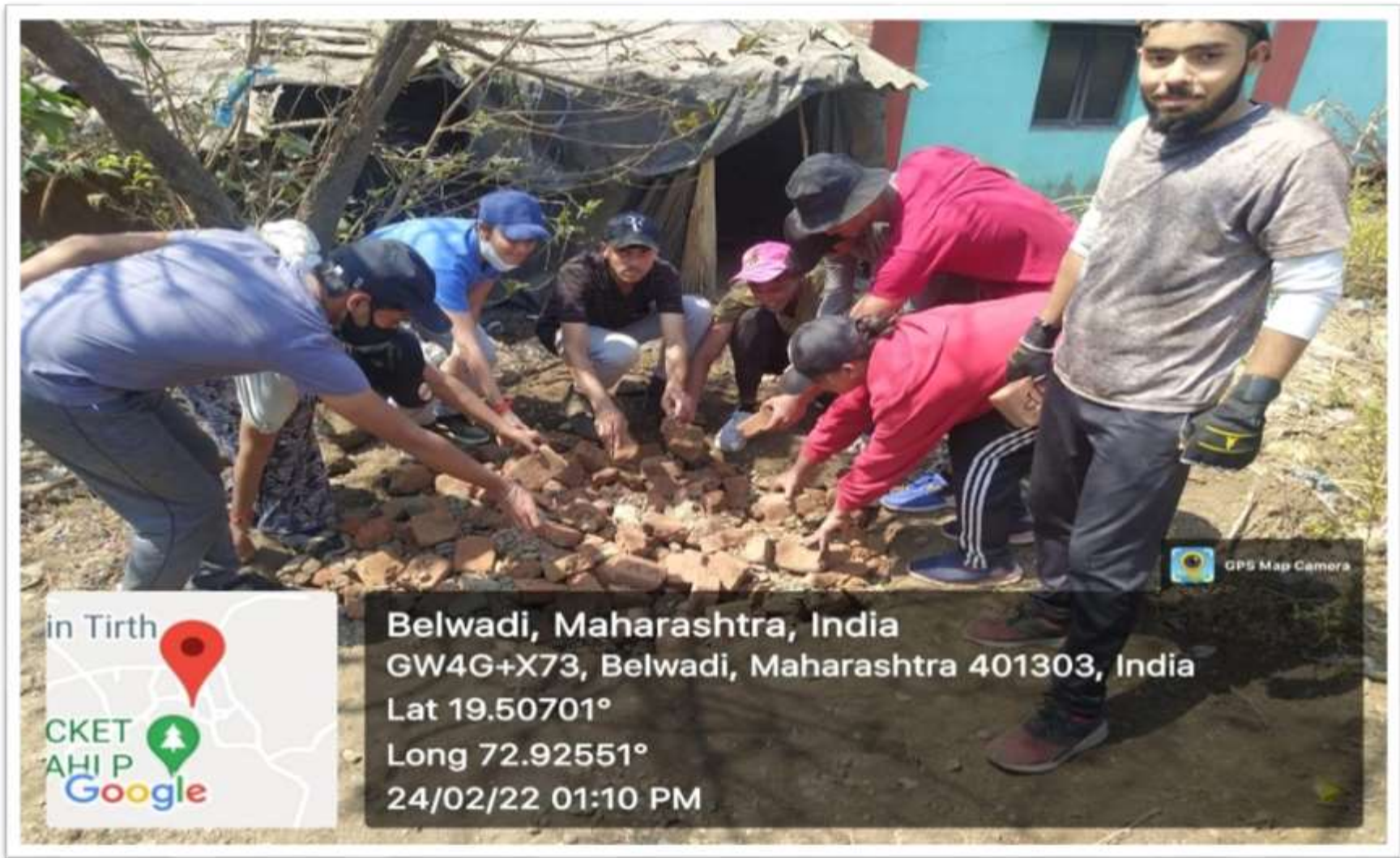
Soak Pit Making at Belvadi
